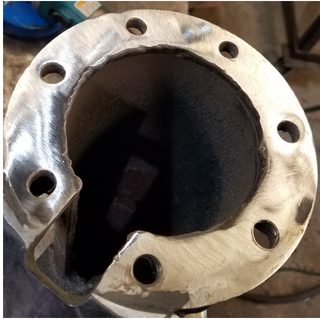
Fig. 4: Flange restored to its original surface profile
